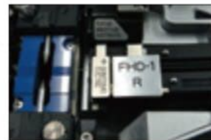
Drop cable splicing with fiber holder system
